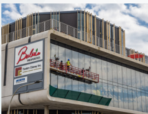
Right: Temporary Suspended Platform being used by Stefanutti Stocs-Axsys-Teichmann JV on the Sentech Tower in Johannesburg
