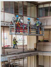
Left: A Temporary Suspended Platform being used by GVK on the Kingsley Centre refurbishment project in Pretoria
